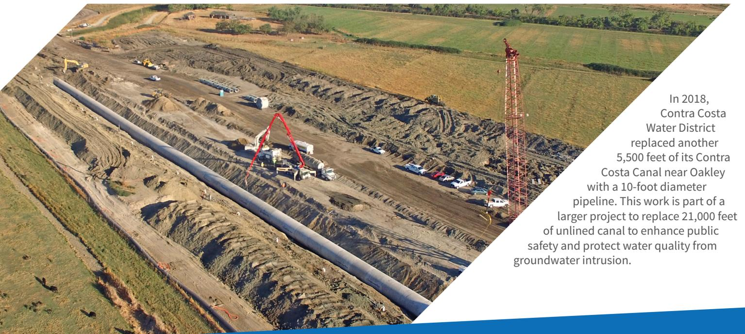
In 2018, Contra Costa Water District replaced another 5,500 feet of its Contra Costa Canal near Oakley with a 10-foot diameter pipeline. This work is part of a larger project to replace 21,000 feet of unlined canal to enhance public safety and protect water quality from groundwater intrusion.
